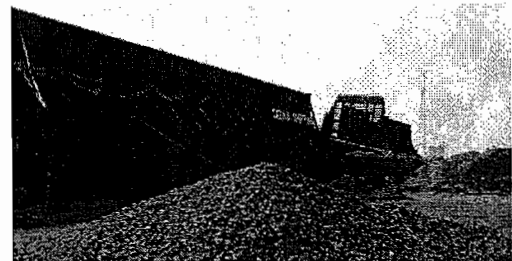
Loading of aggregates onto our barge
